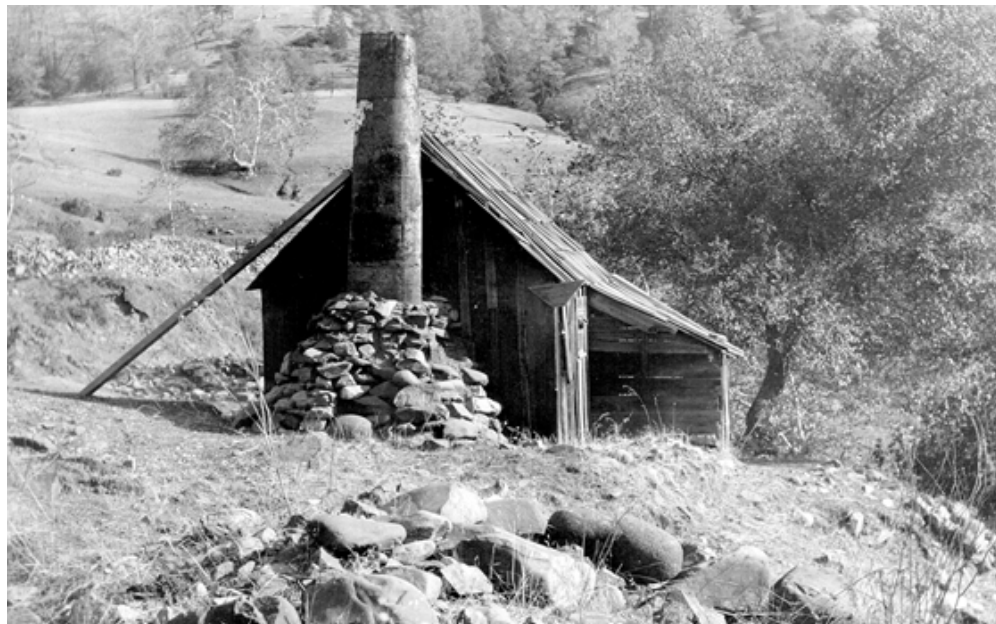
Figure 17: Miner's Cabin near Bidwell Bar, Butte County, 1906. Note the riveted pipe and crude stone used to form a chimney (used with permission, California Department of Conservation, California Geological Survey).
