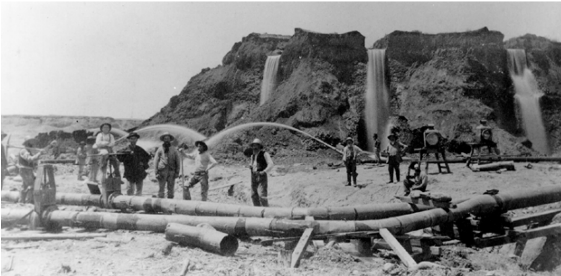
Figure 24: Hydraulic Mining at Michigan Bar, Sacramento County 1860. Waterfalls in background are ground sluices. Locomotive lamps to right of frame are for nighttime flood lights (used with permission, California Department of Conservation, California Geological Survey).
