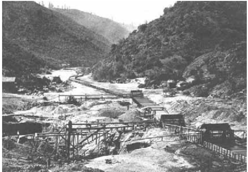
Figure 16: Wing Dams along the Middle Fork American River, 1859 (Courtesy George Wheeldon).
