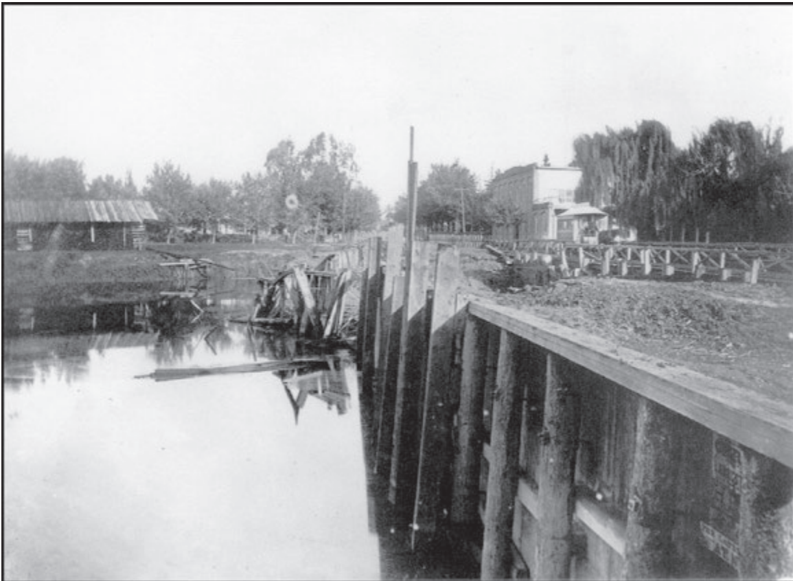
Figure 23. Bulkheads and El Dorado Street Bridge, Miner Channel, ca. 1880, west of project block. (Courtesy of the Bank of Stockton Photo Collection, Stockton, California)
