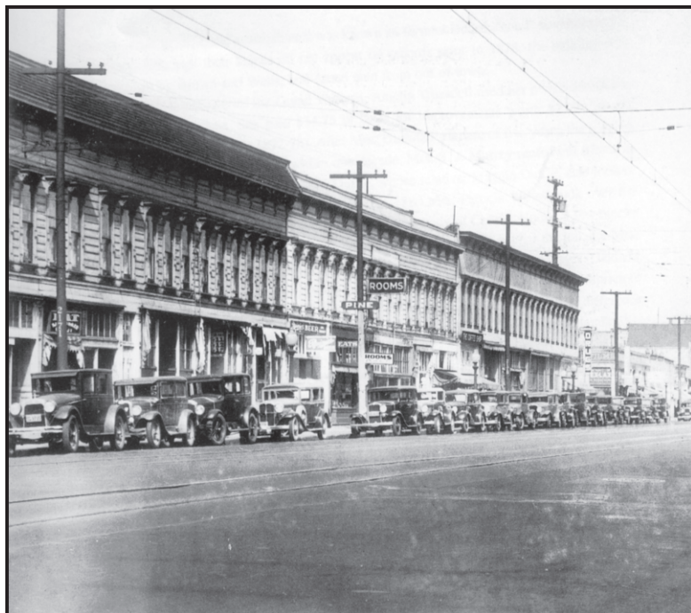
Figure 9.1. Boardinghouse row on Seventh Street, east of Pine Street, in 1940. From left to right, the establishments were the Burlington House Hotel (Bartlett's Hotel), est. 1892; West Oakland Hotel (or House), est. 1869; and Grand Western Hotel (James Block), est. 1873. (Photo courtesy of the Bancroft Library)
