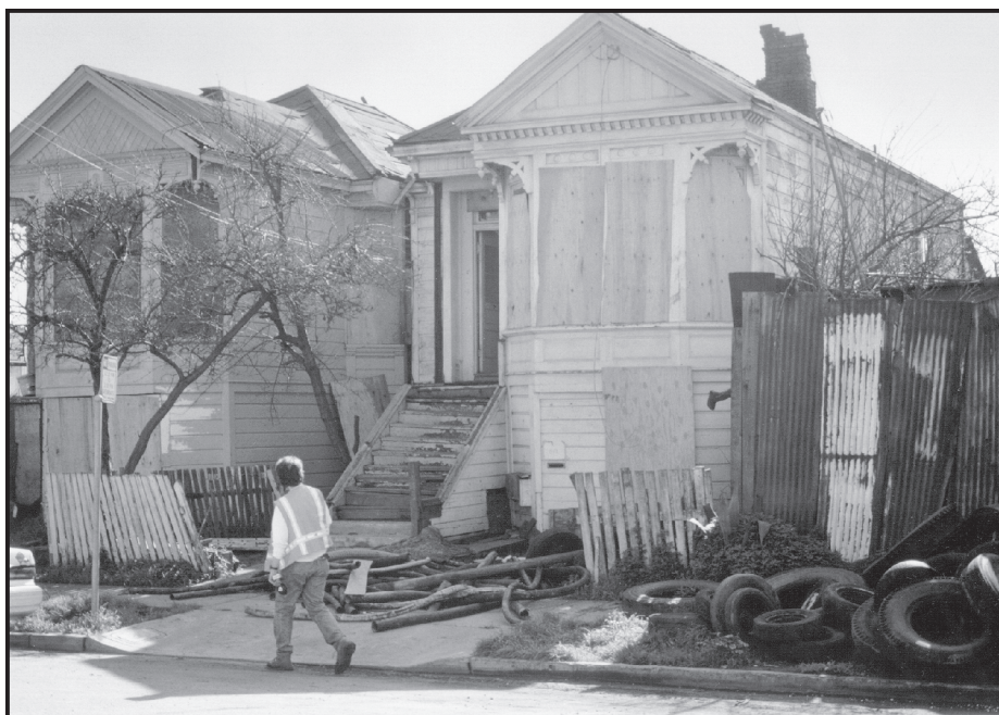
Figure 6.2. Almost-polite house from the mid-1880s. Carpenter Thomas Stevens built three nearly identical Almost-polite houses at 1813, 1815, and 1817 Short Street. His family made their home here, at 1817 Short Street, through 1915. This house was also remodeled and enlarged over the years, prior to being formally recorded for the Cypress Project. The building was moved prior to freeway construction. (Photo credit: Paul Groth)
