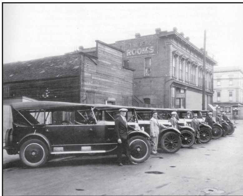
Figure 9.11. The Pullman Hotel around 1912. The hotel can be seen in the background, across Seventh Street; the Mint Saloon operated out of the ground floor. The Buhsen Hotel is in the foreground. (Photo reproduced with permission from Vernon J. Sappers)
