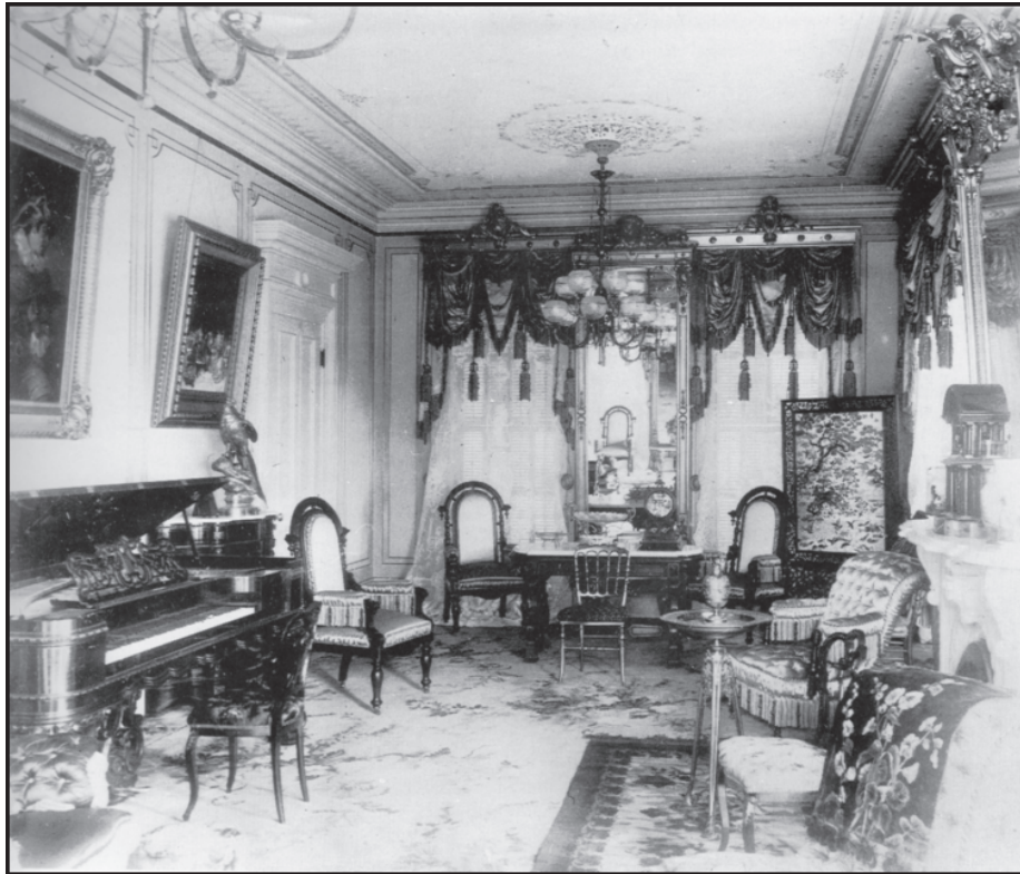
Figure 4.6. The front parlor: an affluent Victorian public space. In the late 19th century, West Oakland's own McDermott house provided a clear model for the exoticized and affluent Victorian parlor. Described as a "front parlor," this room was likely the household's public social space, and it contained choice examples of most of the standard parlor goods. The room had, among other features, oil paintings, a grand piano, silk drapes, Chinese silk screens, and one quite prominent figurine of an eagle or bird of prey standing watch over the room. (Photo reproduced with permission from Vernon J. Sappers)
