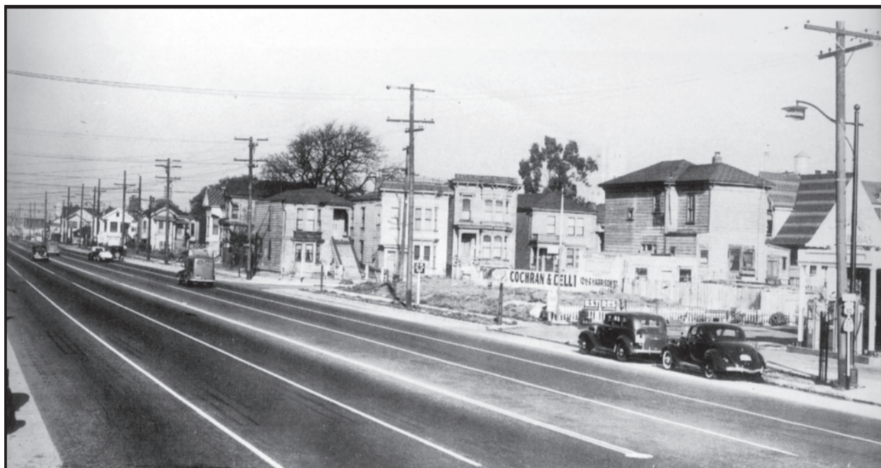
Figure 10.4. End of a neighborhood, 1941. These homes on the corner of Cypress and Eighth streets were removed in 1941 for Peralta Villa. C.L. Dellums recalled the neighborhood's sense of bafflement at what was happening: "The houses that were torn down weren't necessarily dilapidated. The people who were living in their homes... couldn't understand why they wanted to take over their homes for that price when there were places over on Pine and Wood and Cedar in much worse condition. The people had kept their homes up . . . . Their homes were always presentable. But that was the Housing Authority's decision on it, so there was nothing to be done about it" (Henderson 1973:72). (Photo courtesy Oakland Public Library, Oakland History Room)
