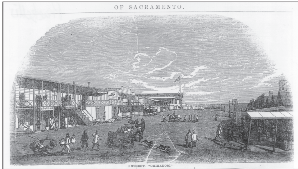
Figure 8.2. I Street "Chinadom," Sacramento. In the mid-1850s, Sacramento's Chinese district centered on I Street between 5th and 6th streets. ASC Archaeologists have conducted excavations on both sides of this street, recovering material associated with various Chinese merchants (Praetzellis and Praetzellis 1982, 1997). (Source: Sacramento Illustrated , Barber and Baker 1855)
