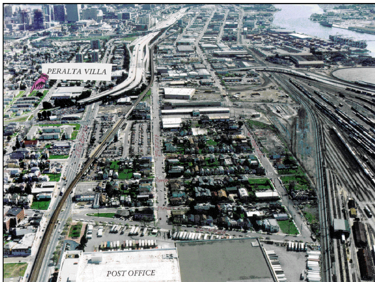
Figure 11.2. The Cypress Freeway and downtown Oakland. From the Seventh Street Post Office complex, we look southeast down Fifth Street to downtown Oakland. The abrupt end of the freeway, just east of Peralta Villa, shows the site of the demolished Cypress structure.
