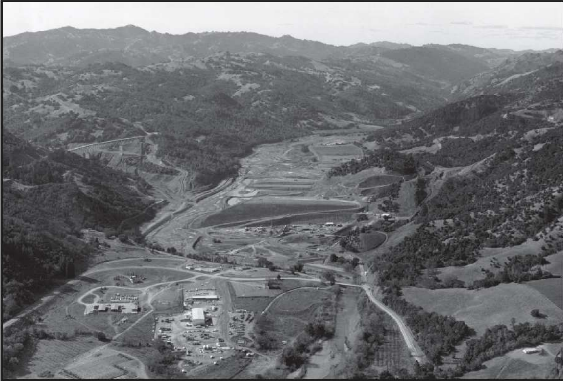
Warm Springs Dam under construction circa 1979; Rockpile Road Bridge crosses Warm Springs Creek at middle left.
