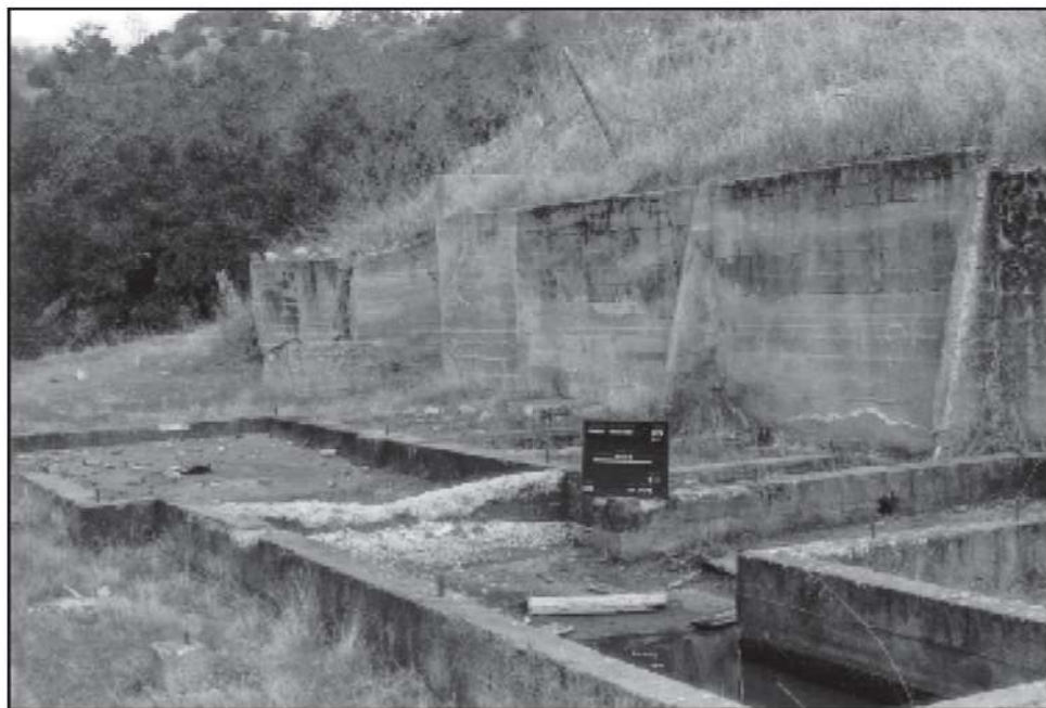
Foundations of the Skaggs Springs quicksilver mine, 1976
