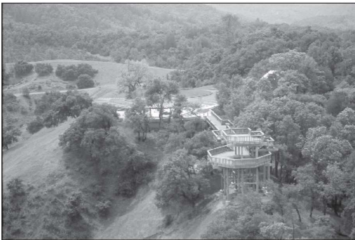
Overlook above Warm Springs Dam
