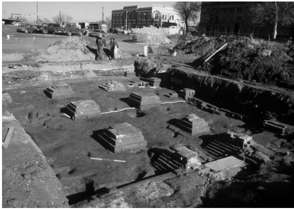
Figure 95. Square brick piers supported the wooden floor joists of commercial buildings. High real estate prices encouraged merchants to construct multistory buildings in which commercial and residential functions were separated according to floor (Photograph by ASC, Sonoma State University).
