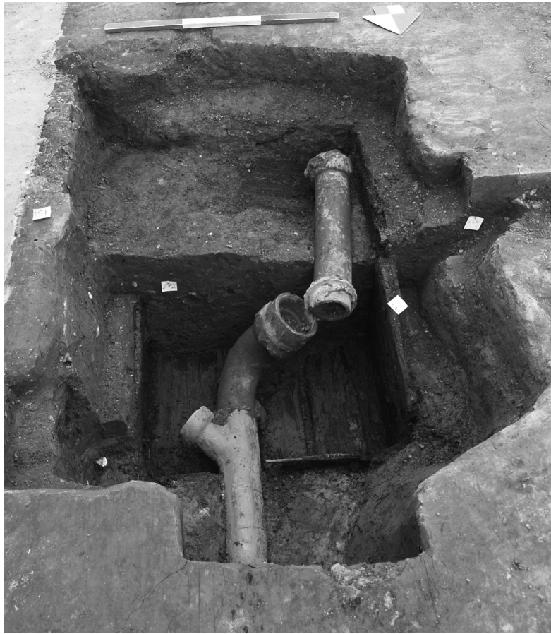
Figure 94. Redwood drains, Heinlerville, Santa Clara County, circa 1880s. To prevent construction of Heinlerville in the 1880s—a Chinese and then Japanese community—local officials insisted that the development have individual sewer connections. The redwood drains soon gave out and by about 1906 were replaced with a modern system of ceramic pipes plumbed into the main sewer (Photograph by ASC, Sonoma State University).
