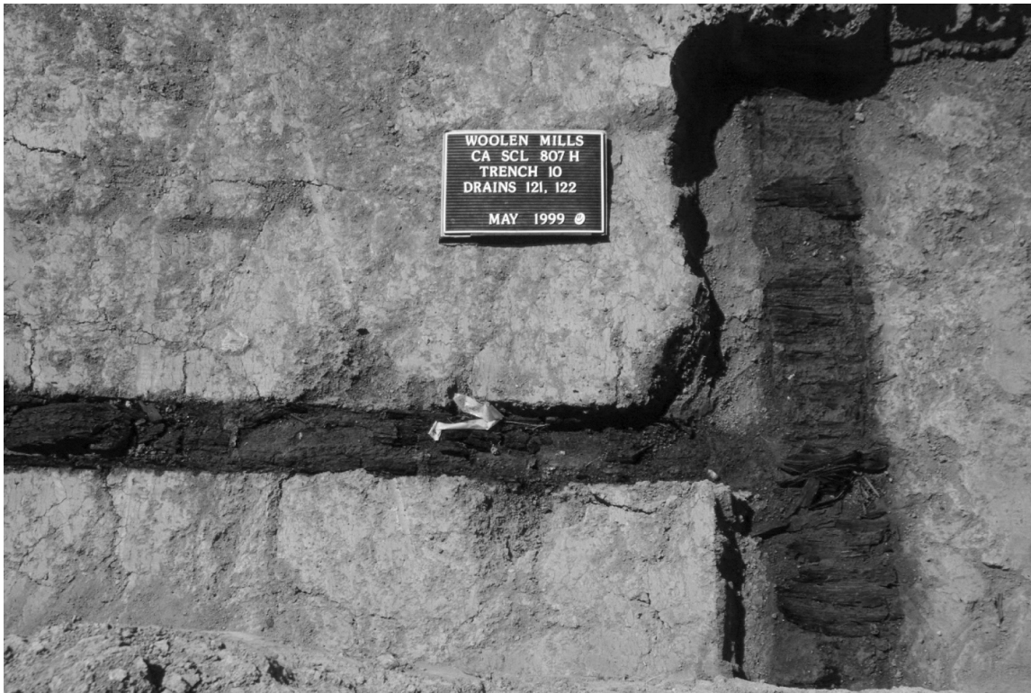
Figure 83. Redwood box drain, Woolen Mills Chinatown, San Jose, circa 1887 (Photograph by Jerry Doty, KEA Environmental).
