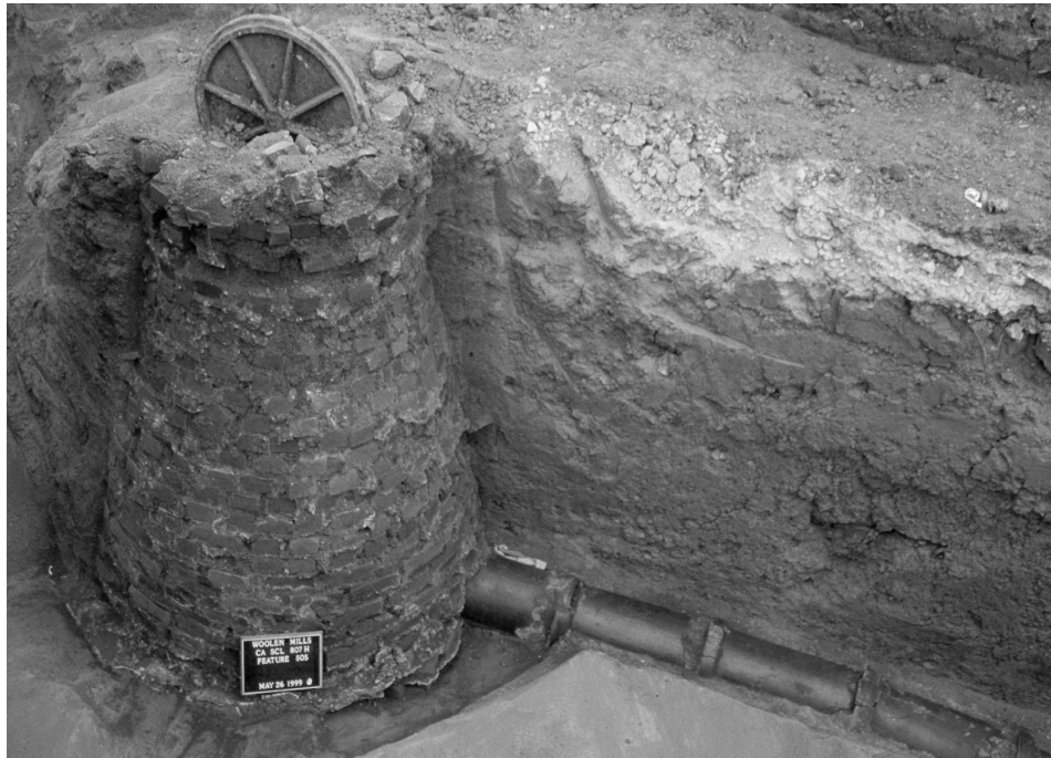
Figure 82. Brick vault and stoneware sewer pipe, Woolen Mills Chinatown, San Jose, circa 1887 (Photograph by Jerry Doty, KEA Environmental).
