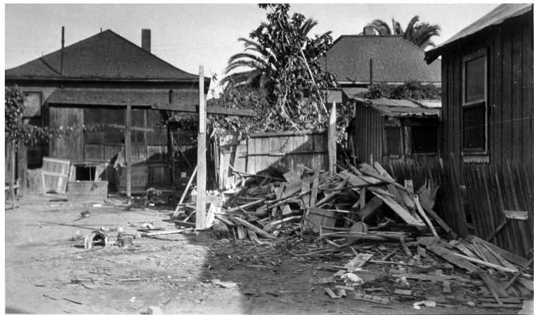
Figure 37. Backyards of a suburban neighborhood, Santa Clara, California, circa 1910. Note the trash, lumber, and lack of sanitation; such conditions were prevalent in towns throughout the state during the early-20th century (Courtesy of The Bancroft Library, University of California, Berkeley).
