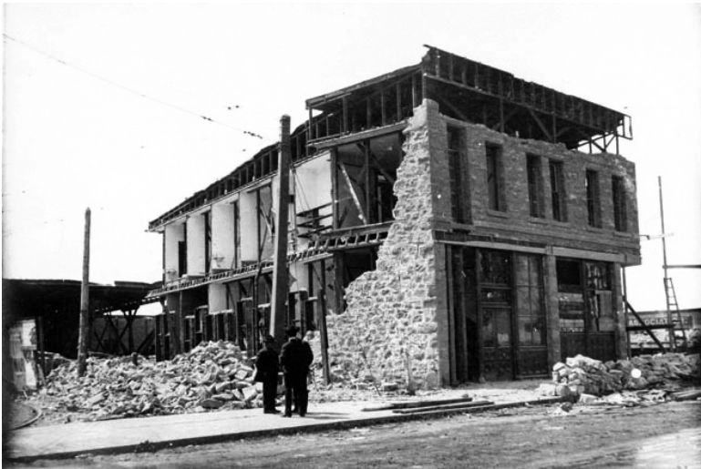
Figure 45. Earthquake damage to a reinforced stone-masonry building in Santa Rosa, 1906 (Courtesy of The Bancroft Library, University of California, Berkeley).
