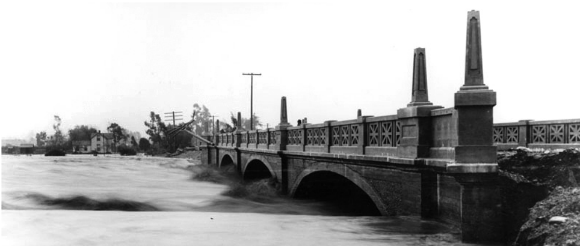
Figure 29. East Chapman Avenue Bridge, Orange, California, threatened by Santa Ana River floodwater, 1916 (Courtesy of Orange Public Library, Orange).
