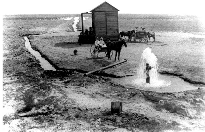
Figure 34. Artesian Well, Lower San Joaquin Valley near Bakersfield (Carl Watkins Photograph, Courtesy of San Joaquin Valley Library System).
