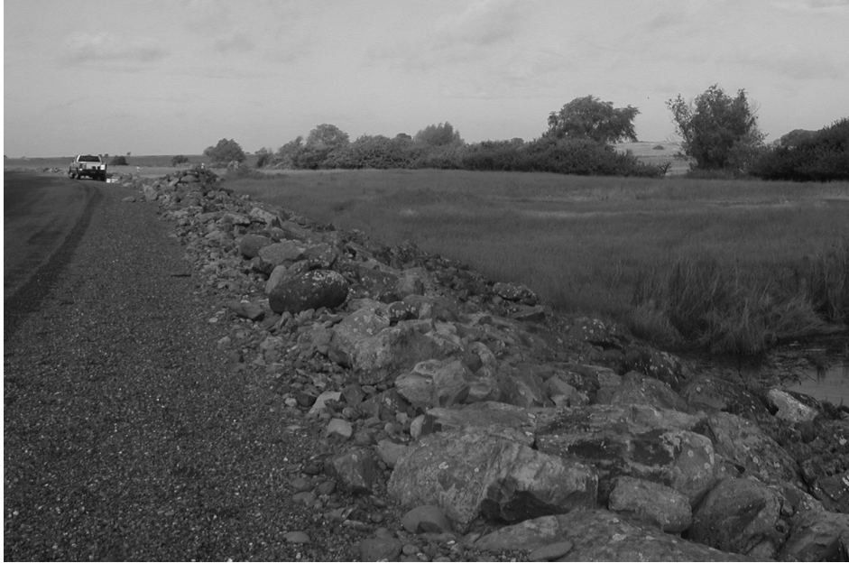
Figure 81. Levee road, Oroville vicinity. The proclivity of early Californians to build towns on floodplains was mitigated by building levees whose tops were used as roads (Photograph by ASC, Sonoma State University).
