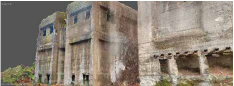
Model of the Research Mine Furnaces (Lake County) created with Agisoft Metashape from data collected with a DJI Mavic Pro.
