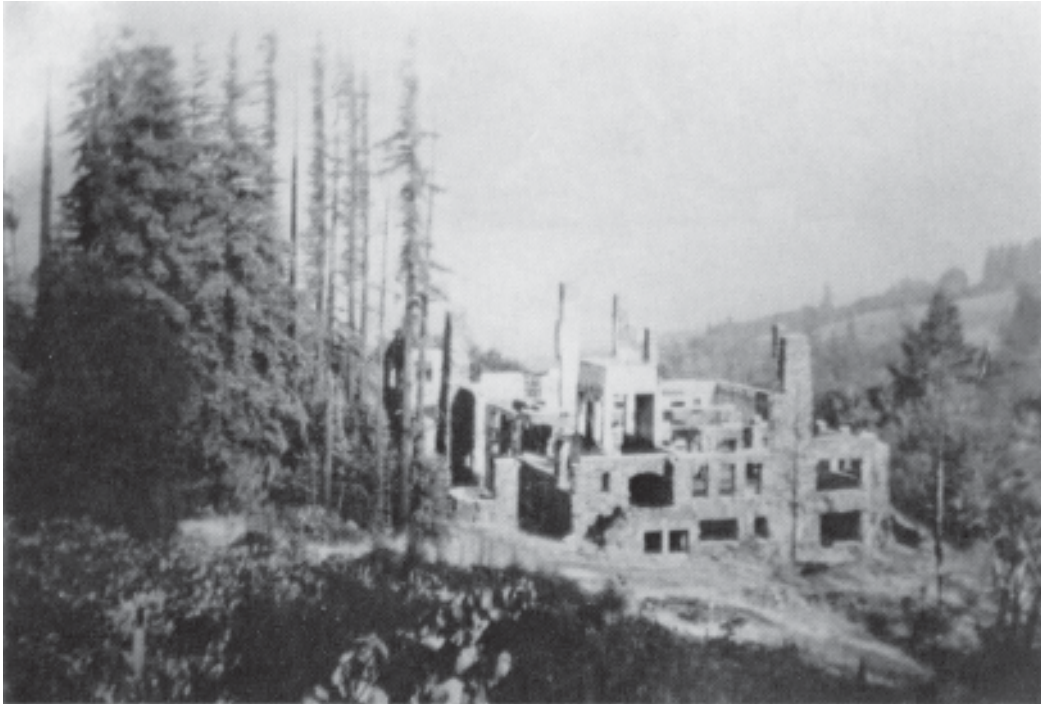
FIGURE 9. The Wolf House ruins. The cause of the fire was never determined. (courtesy of the California Department of Parks and Recreation.)
