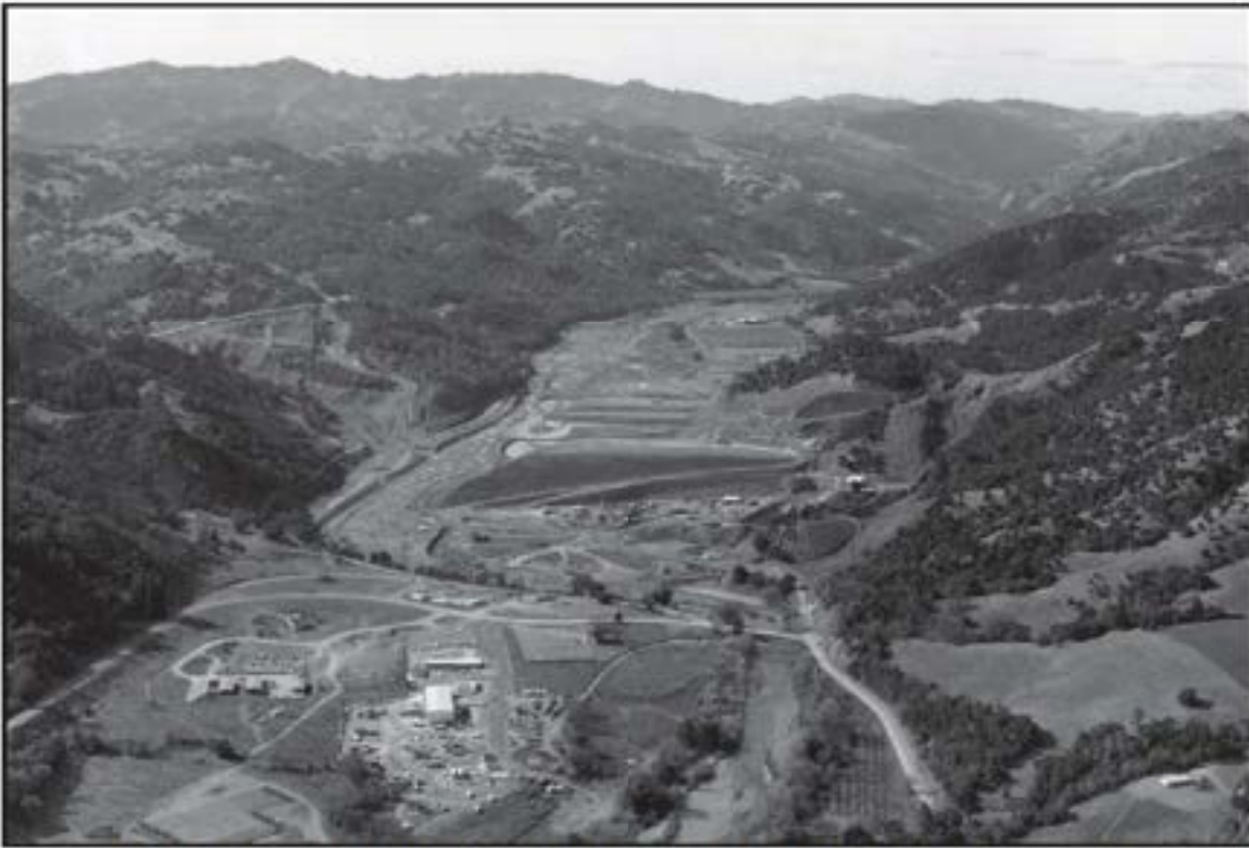
Warm Springs Dam under construction circa 1979; Rockpile Road Bridge crosses Warm Springs Creek at middle left.
