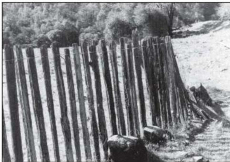
Split-stake fencing in the Dry Creek uplands (photo by Karana Hattersley-Drayton)
