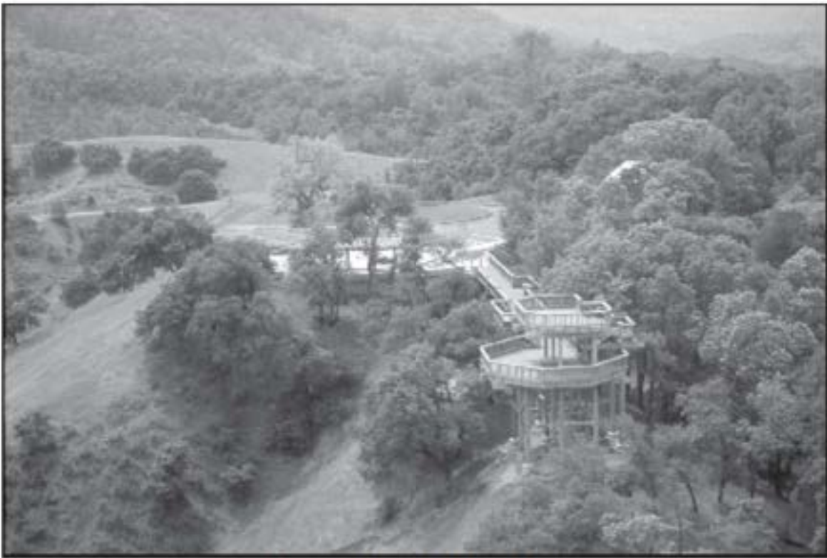
Overlook above Warm Springs Dam
