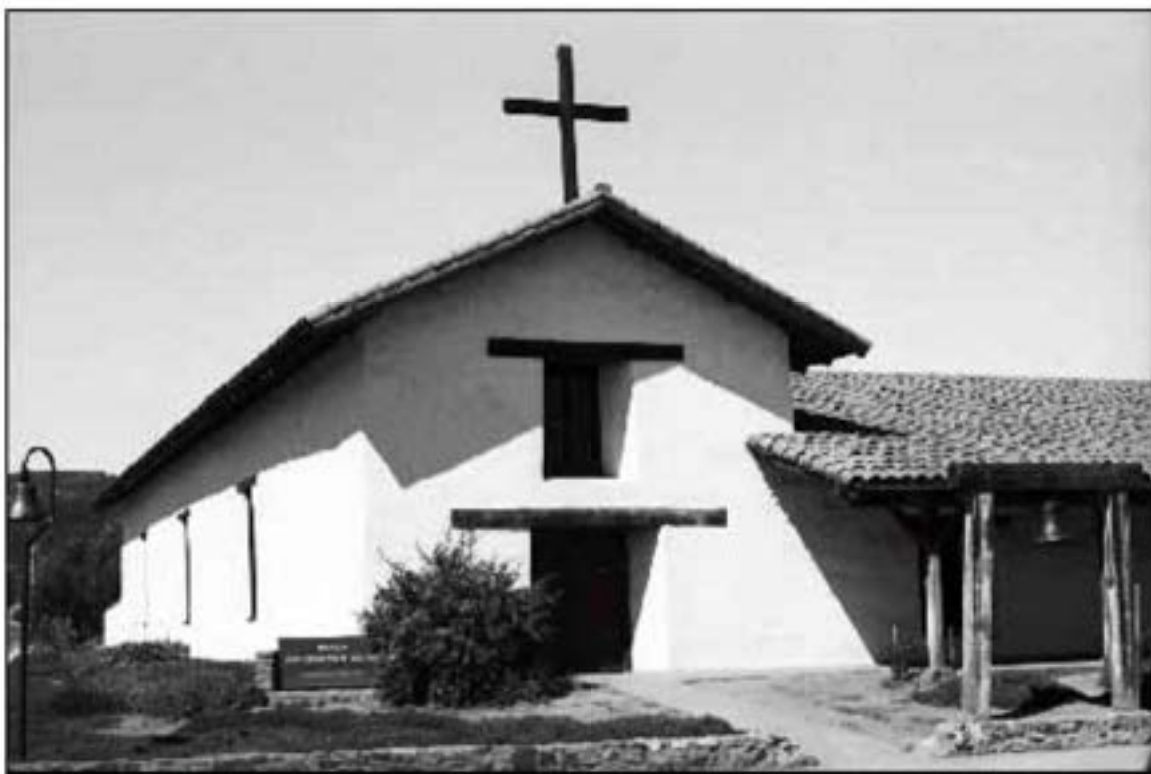
Mission San Francisco Solano de Sonoma, established 1823 [restored]
