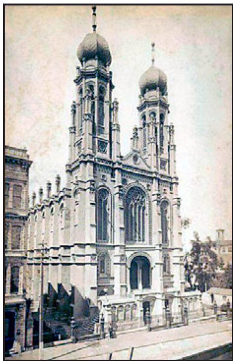
Figure 8.4. The Sutter Street Synagogue. This 1866 building was home to Congregation Emanu-El. The building is an interesting marriage of church-like architecture and subtle Jewish symbols. The Magan Dovid (Star of David) is displayed significantly above the line of sight, while the twin domes evoke the crowns ( keterim ) used to decorate the etz chaim , the wooden handles of the Torah scroll. (Photo courtesy of the California History Room, California State Library, Sacramento, California)
