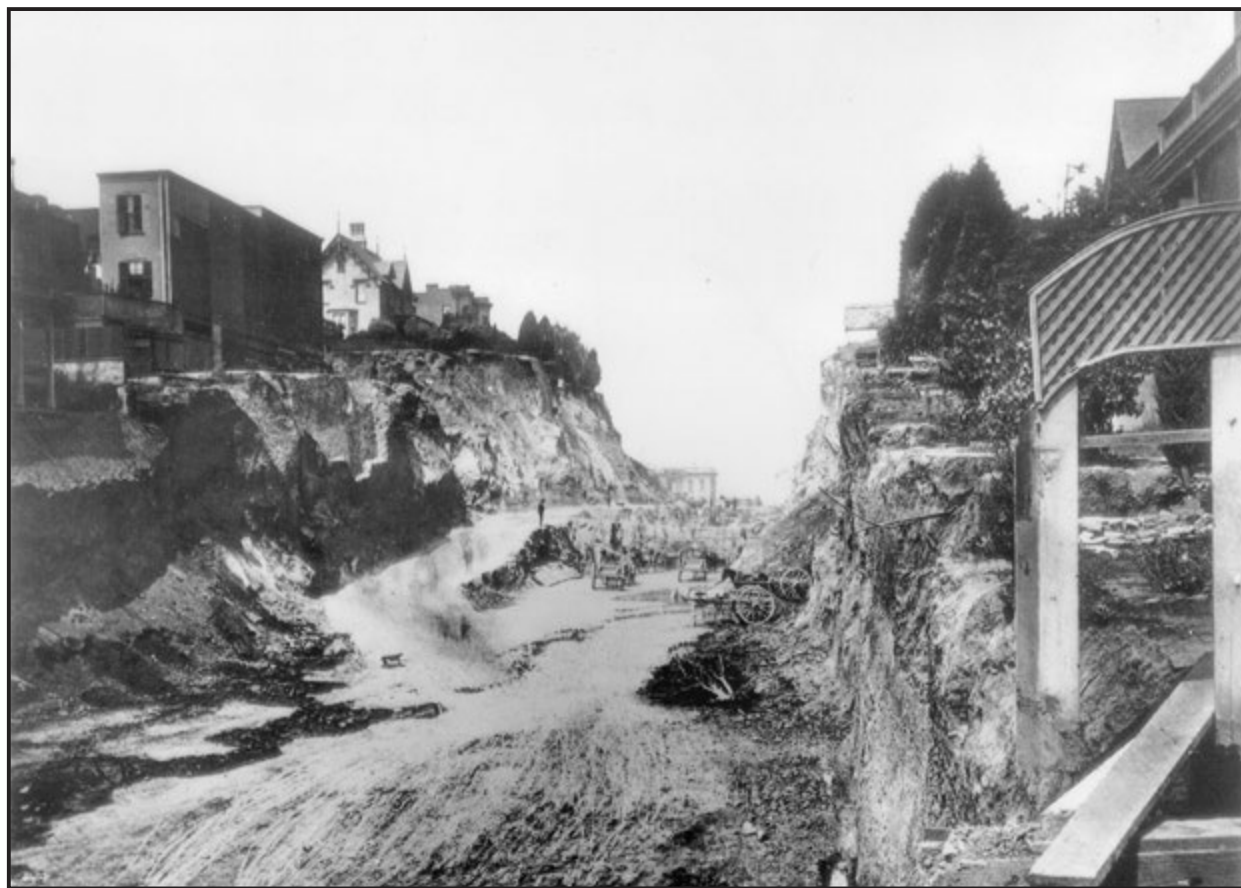
Figure 10.4. Second Street Cut in Progress, Looking Northwest from Bryant Street, 1869. Two hundred and fifty teams of horses and wagons, together with five hundred men, worked from April through November trying to shore up the cut as avalanches, "sometimes fatally interrupted" grading (SF City Directory 1869-1870:16). The peaked-roof and gabled house at the west corner of Harrison and Second Street eventually fell into the ditch below, as did the house across the street (Photo courtesy of the Bancroft Library, University of California Berkeley: 1905.07052--PIC).
