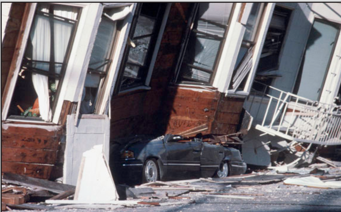
"Loma Prieta, California, Earthquake October 17, 1989. San Francisco. An automobile lies crushed under the third story of this apartment building in the Marina District [USGS Open-File Report 90-547]." (Photo by J.K. Nakata, USGS)
